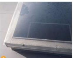
1. Adhesion issue at waterproofing membrane
