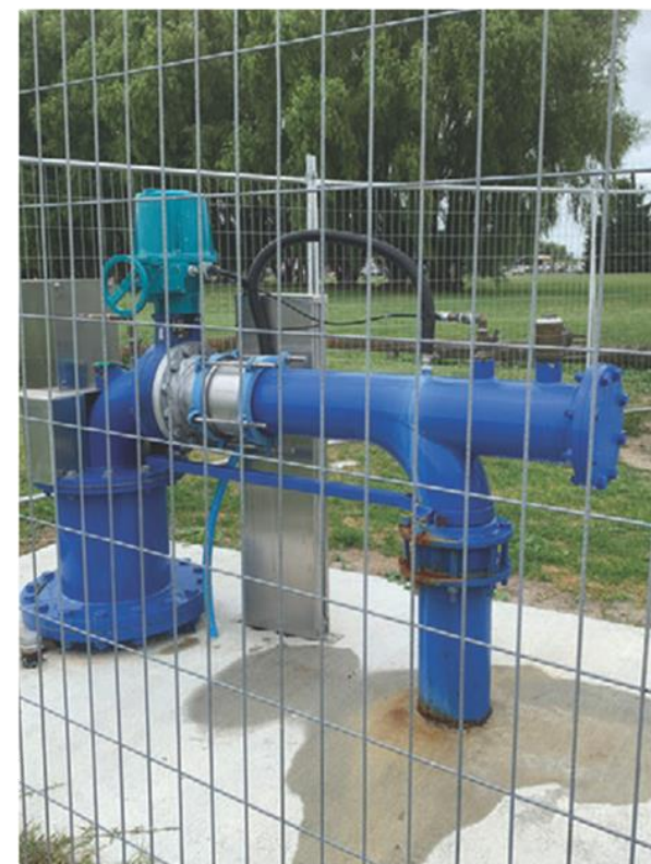
Figure 9 New bore at Tareha Park. This draws water from the Heretaunga Plains aquifer and supplies water to local residents.
