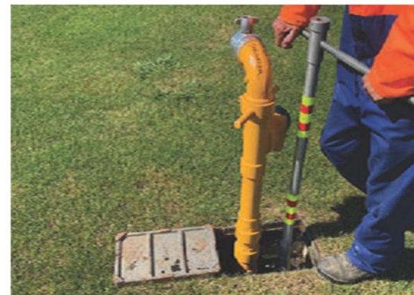
Figure 38 Non-return valve connected to a fire hydrant at Petane War Memorial Reserve to prevent backflow and contamination risk.
