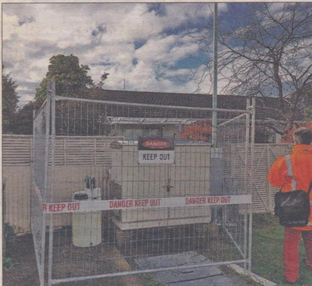
CHLORINE SOURCE: The secure chlorine dosing site in Taradale, which injects chlorine into the reticulated system 24 hours a day, for as long as is needed.
