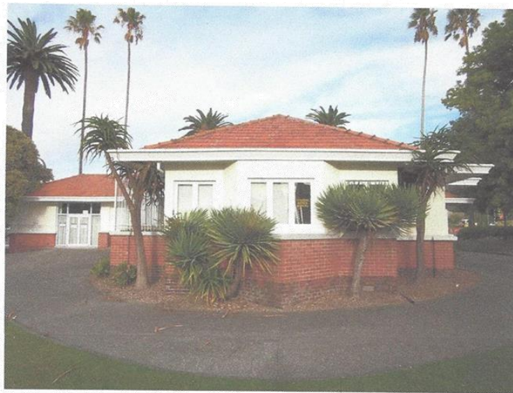
Figure 7: Front (east) including angled planter box that once formed part of the verandah but has since been closed in. Note the rusticated brick courses at the bottom which was preserved from the original design after the earthquake.
