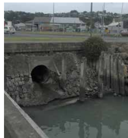
Top. Existing. Outlet (broken)discharging Meeanee Quay catchment direct to Inner Harbour with no water quality treatment
