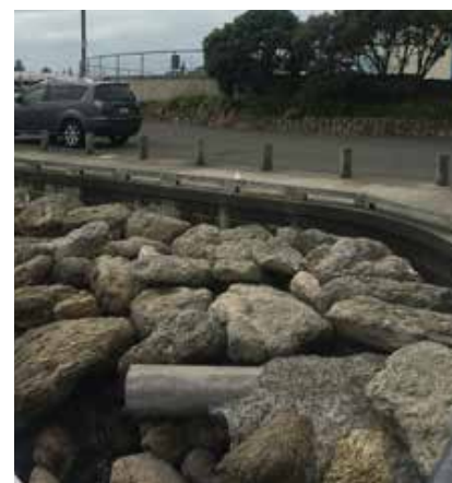
Middle. Existing. Large outlet discharging rail yard catchment direct to Iron Pot with no water quality treatment.
