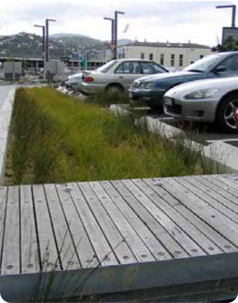
Right. Low impact stormwater treatment options - planted raingardens, mechanical filters.
