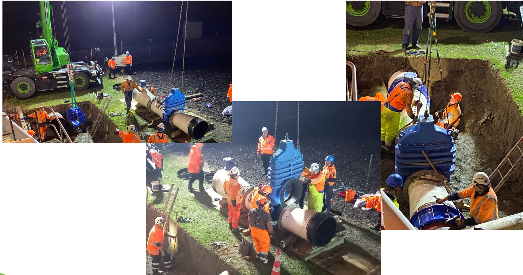
Replacement of the inlet valve from Latham Street
