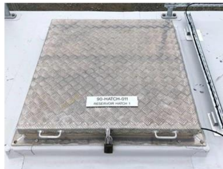
Figure 7 - Hatch on Tironui reservoir which is covered with roof membrane (June 2020)
