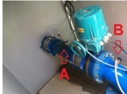
Figure 13 - A) Typical chlorine dosage entry point and B) Raw water sampling point
