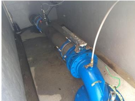
Figure 2 - Coverdale (C1) bore head in refurbished dry chamber (as on 16 Jan 2018)
