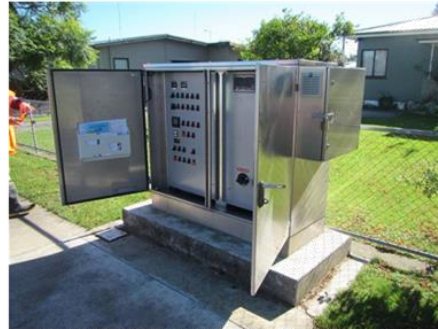
Figure 3 - Typical bore electrical control cabinet (November 2017)
