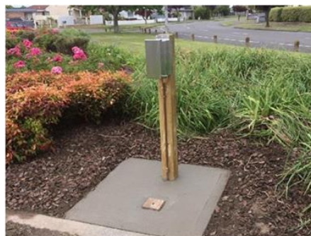
Figure 11 - 9 Tait Drive - typical NCC reticulation sampling tap (January 2018)
