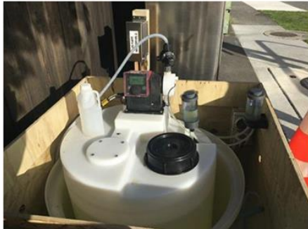
Figure 12 – Typical chlorination setup, T7 bore (June 2020)
