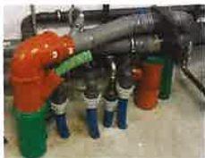
Example for pressure lines with Plasson screw connection and empty conduits
