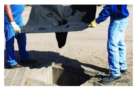
Witches Hats – Filtering storm water at the sump to remove debris, sediment and contaminants from the system.
