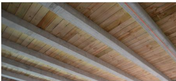
Exposed Stalhton Rib & Infill
