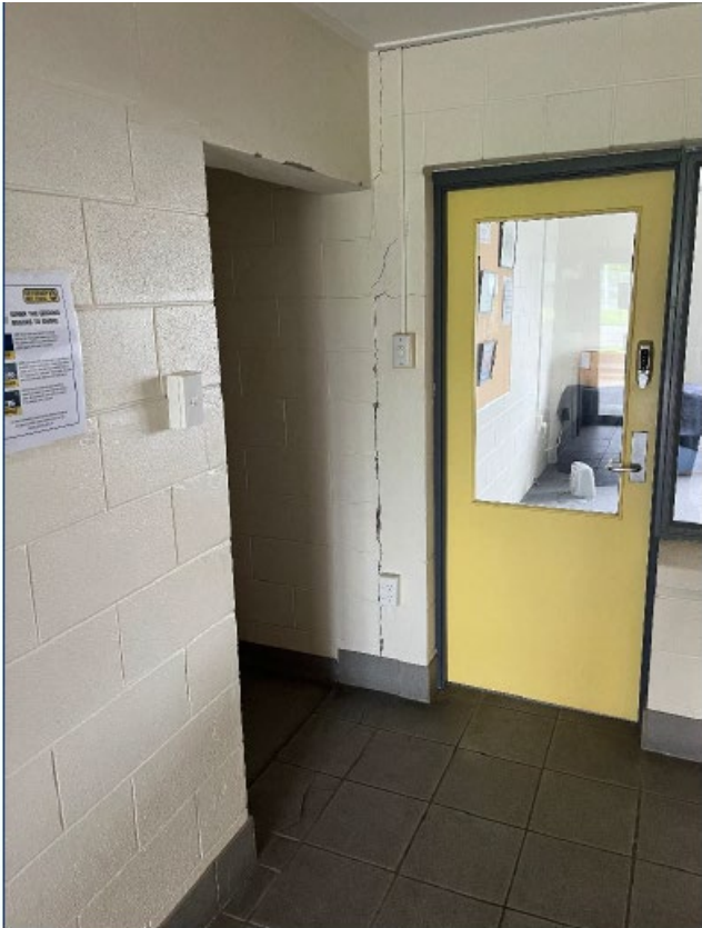
View of crack in internal wall
