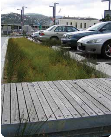
Right. Low impact stormwater treatment options - planted raingardens, mechanical filters.
