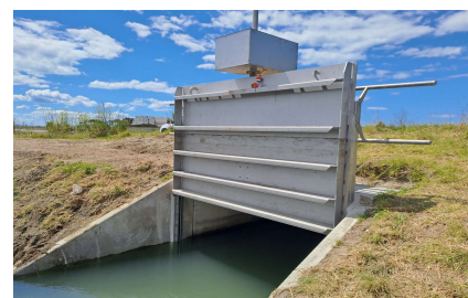
Purimu channel stormwater gate installation work in progress
