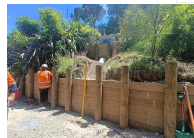
Lighthouse Road Storm water works completed
