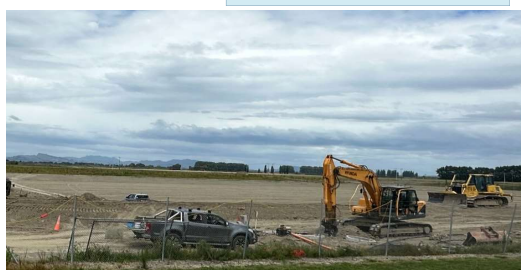
WWTP Cell 3 Construction work in progress
