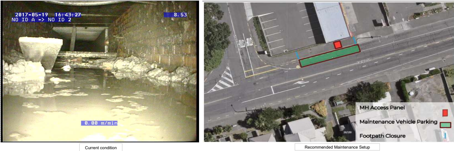
Carlyle Street stormwater culverts have reduced capacity due to silt accumulation. The proposed project involves installing access hatches to enable future cleaning, maintenance, and inspection.
