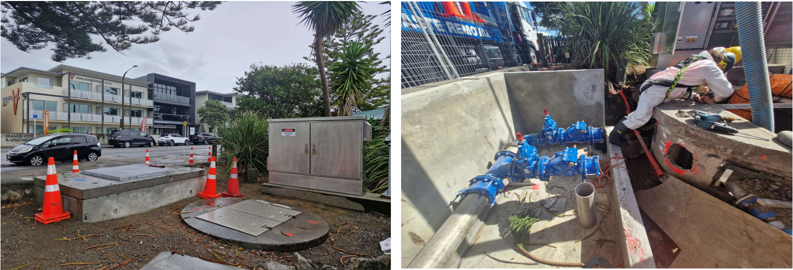
Upgrades to the Stafford Street Pump Station included a new pump and pipework to improve resilience, along with replacement of deteriorated valves, the chamber, and installation of a flow meter
