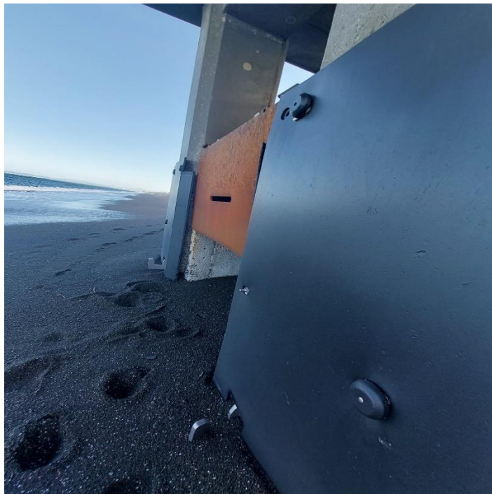
Figure 5: Abrasion found on the metal plate
