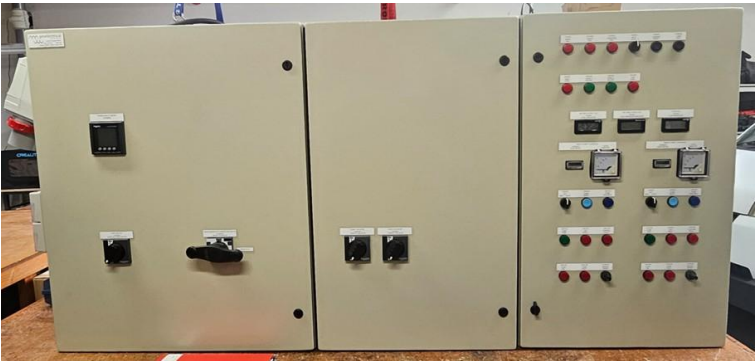
Constable Crescent Waste water Pump Station upgrade work completed under NCC new SCADA system
