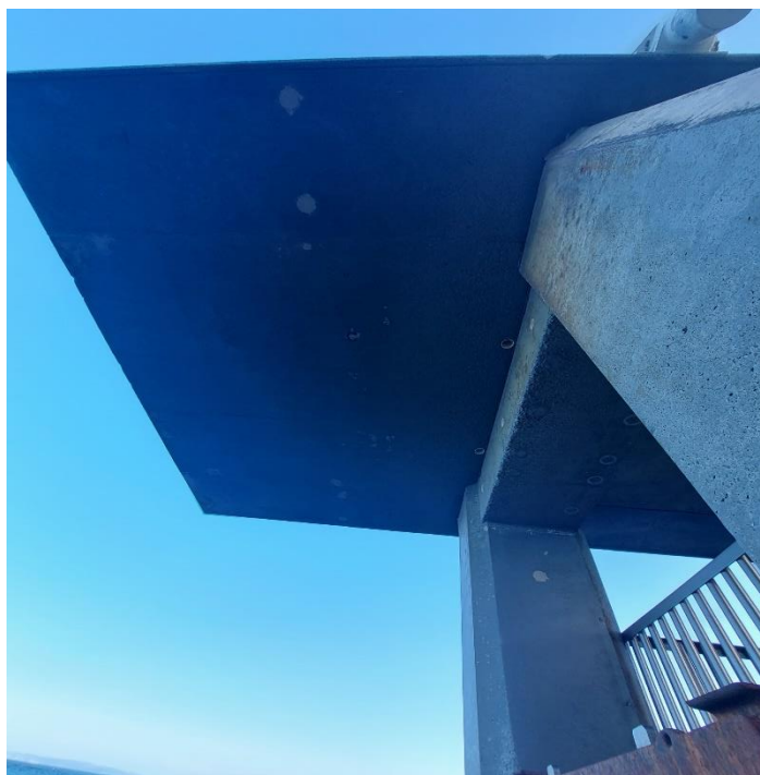
Figure 6: Scouring can be found on the concrete surface due to the waves hitting
