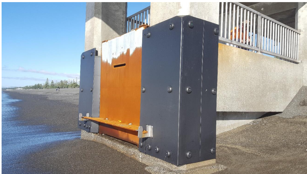
Figure 9 HDPE Shields at the side
