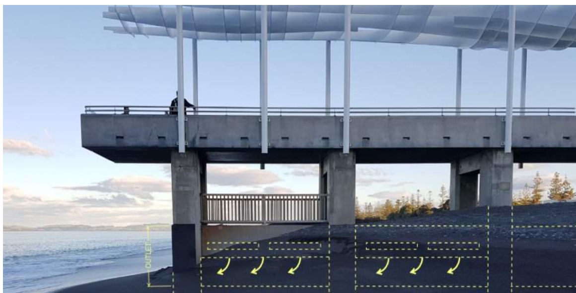
Figure 2 June 2021 showing all side orifices blocked
