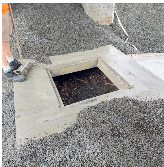
Figure 4: Extend of beach material getting into outlet
