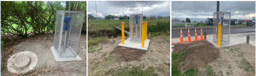
The Air Valves on Watermains at Eriksen Road, Prebensen Drive and Taradale Road
