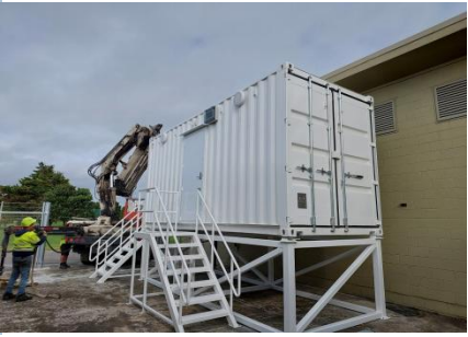
New SCADA Server Container Installed at 286, Te Awa Avenue
