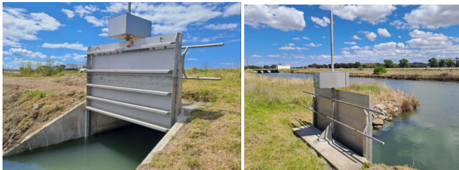
Purimu Channel Stormwater Gate Installation Work
