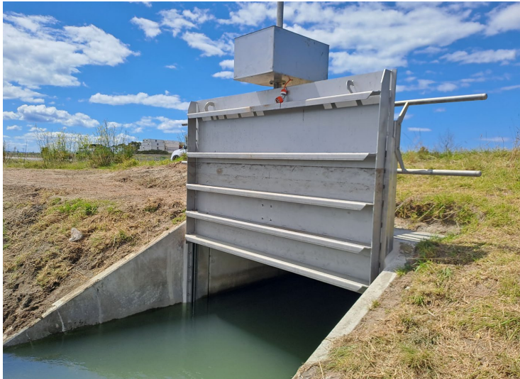
Purimu Channel Stormwater Gate Installation Works.
