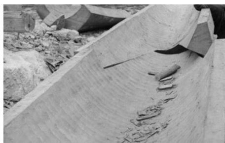
Fig 2.1.2 Haumi joint under construction
